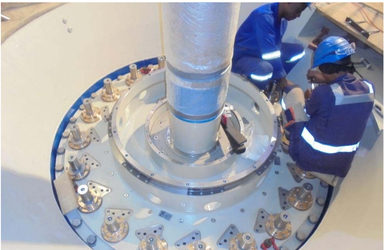
Photo: Assembling of the new turbines at Mwadingusha in progress.
